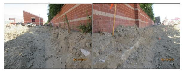
The plan was to excavate and create a Mouse Trap (an underground confined space with tunnels for the trainees to practice lugging equipment around and to create real-life dire situations they will face in the field - hence the term "mouse trap"). The excavation for the Mouse Trap required an approximately 10-feet-high steep slope next to the wall that was planned to remain open for about four to six weeks while the Mouse Trap was constructed.
