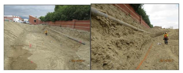
No movement of the wall or the pipe was observed during the excavations, and the sides of the excavation were stable throughout the excavation activities.
