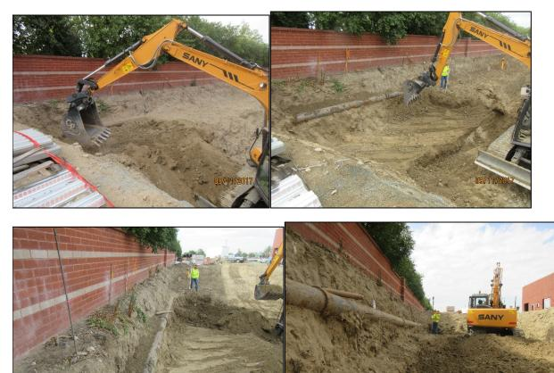
Another site visit took place a couple days later to observe the excavation and to observe the progress of construction. The excavation was extended an additional 18 inches deep to place forms for the proposed wall footings.
